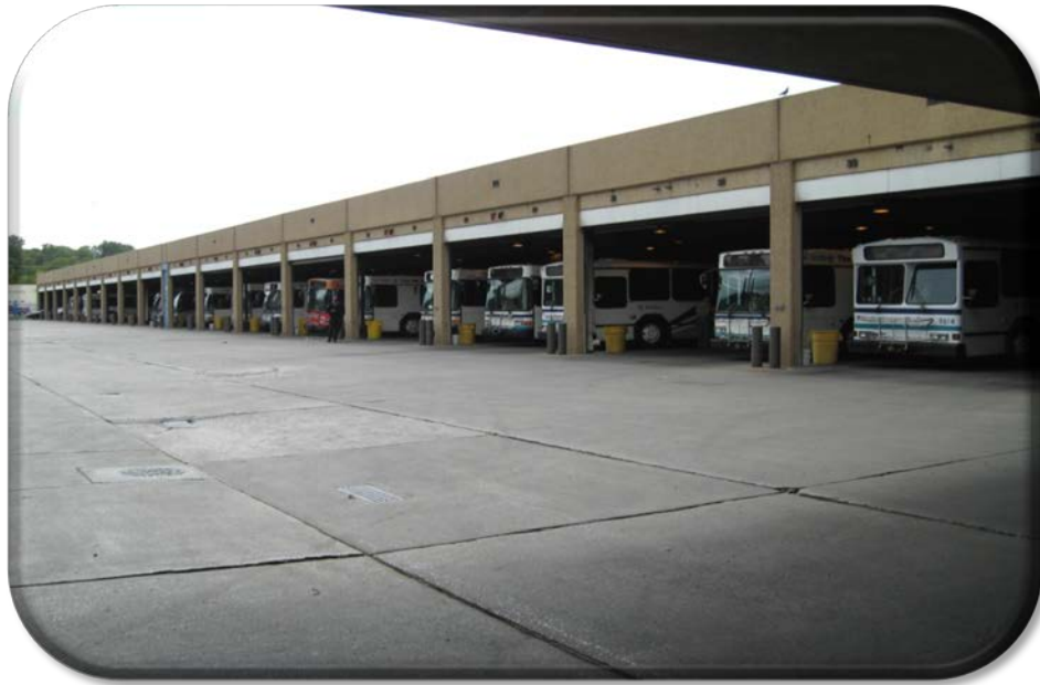
Figure 3: View of East Side of Vehicle Storage Building
