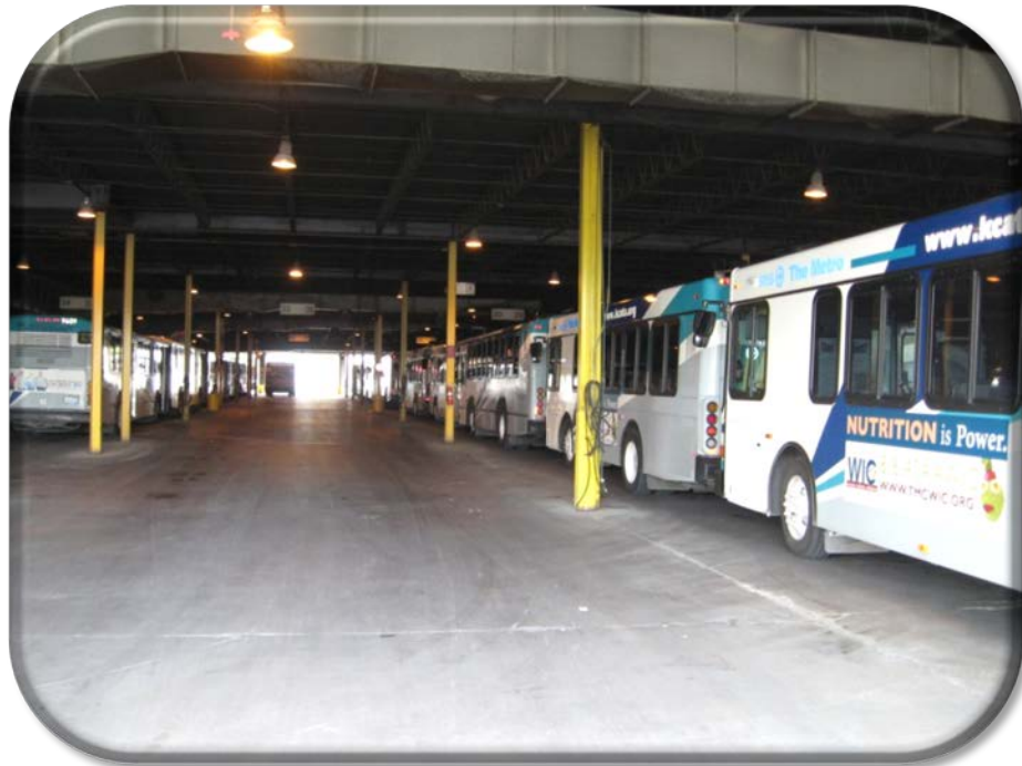
Figure 4: View Inside of Vehicle Storage Building (West Entrance facing East)
