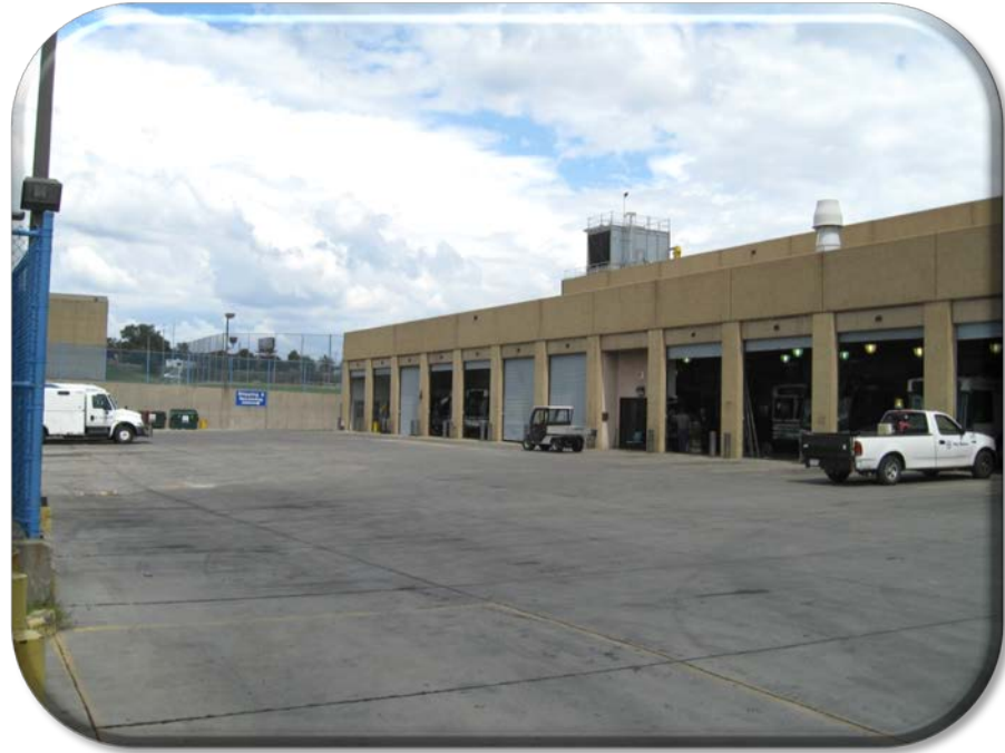
Figure 6: External View of Vehicle Maintenance Building (West Side)
