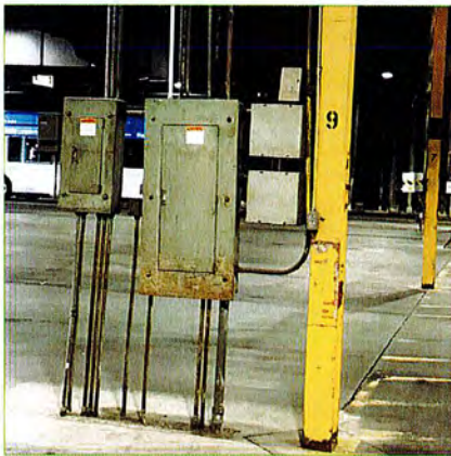
Panel B (480V) and Panel D (208V)
