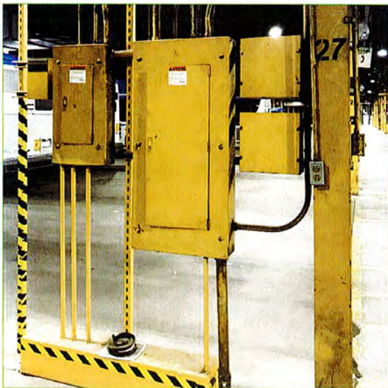
Panel A (480V) and Panel C (208V)
